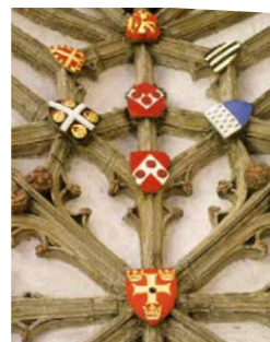
Fig. 2 Vaulted ceiling England, Canterbury Cloister 15th century
