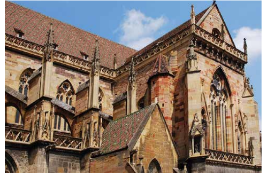
Fig. 1 Nave and South Transept of St Martin's France, Colmar c. 1250 – 1300
