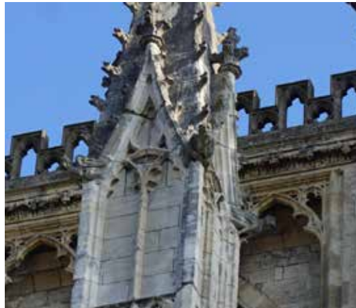
Fig. 1 Lady Chapel buttress pinnacles, with gargoyles visible at the base c. 1361–73 York, Minster
