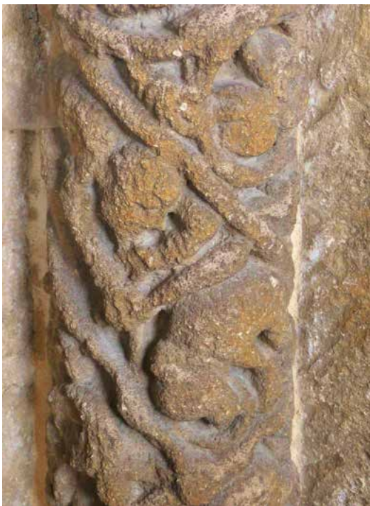
Fig. 4 Detail of the 'Prior's Door' England, Ely Cathedral c. 1120-40
